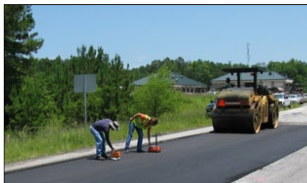
Figure 1 Monitoring field compactability.
