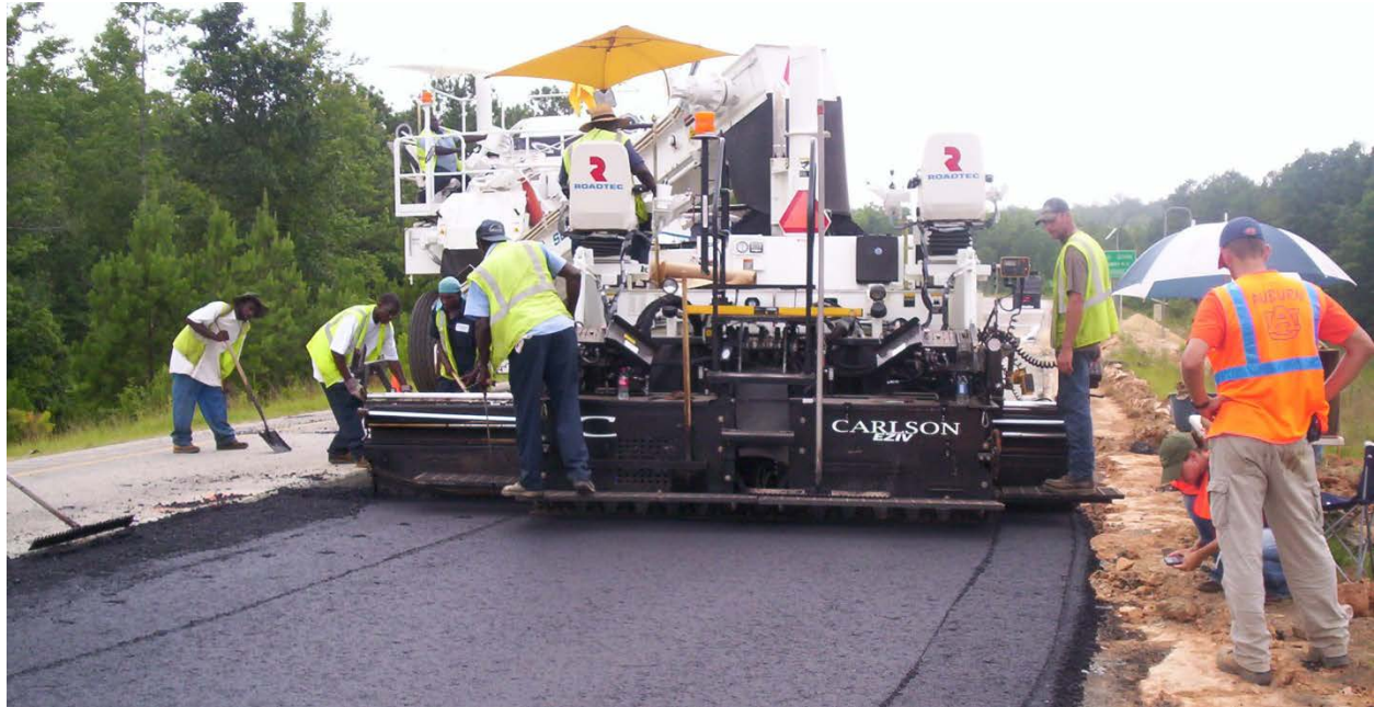
Figure 1.3 Paving the Surface Layer of a Test Section on the 2009 NCAT Test Track
