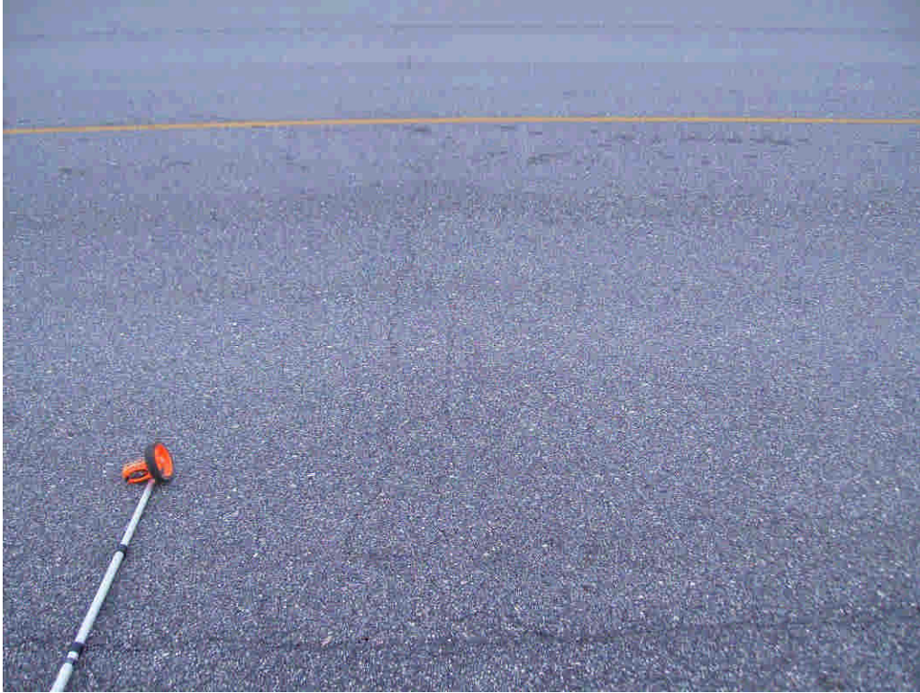
Figure 23: Reflective Cracking
