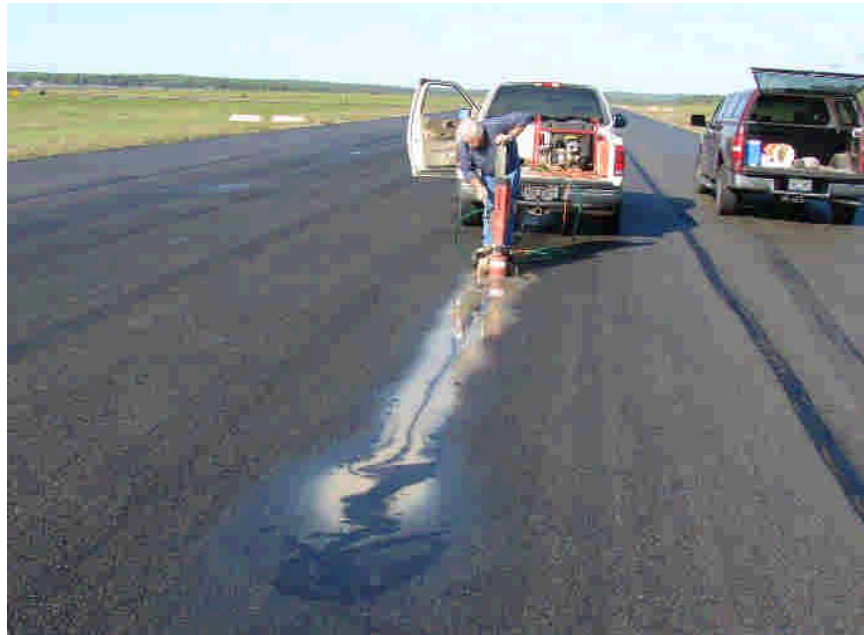
Figure 18: Core Water Collecting in Rut
