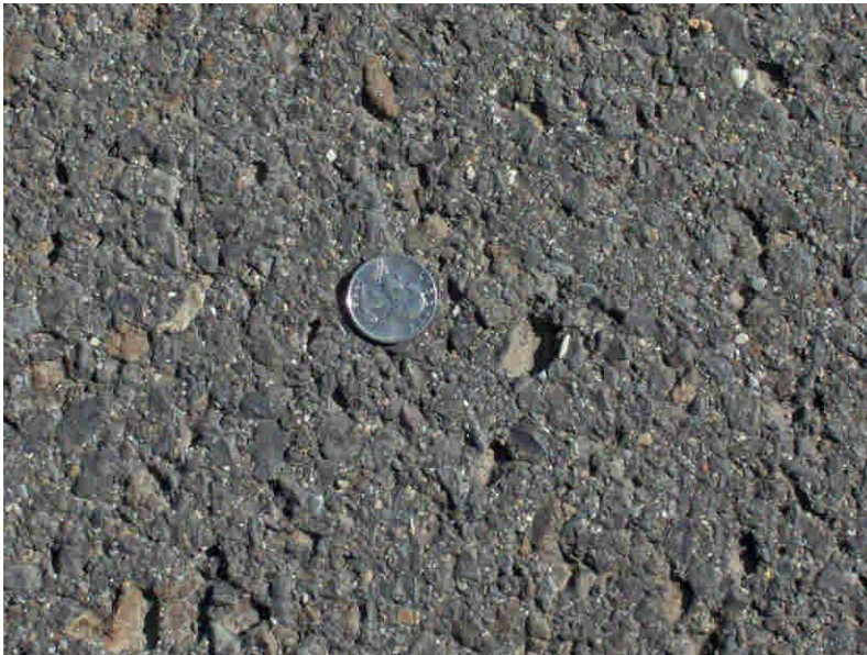
Figure 36: Typical Raveling
