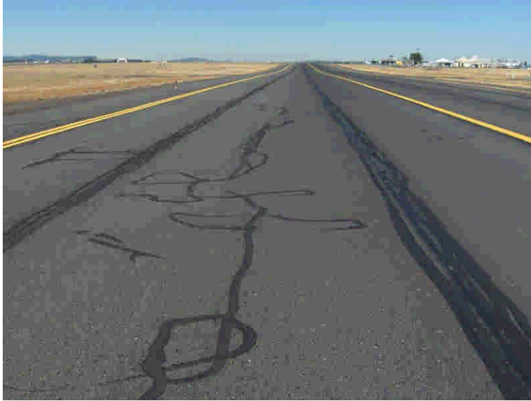
Figure 37: Typical Crack Sealing
