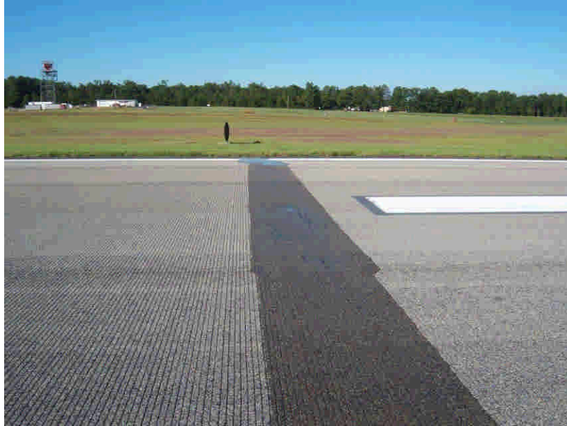
Figure 30: Proper Evacuation of Core Water by the Pavement Grooving and Cross-Slope
