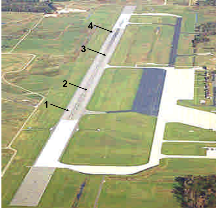
Figure 24: Aerial View of Airfield with Core Locations
