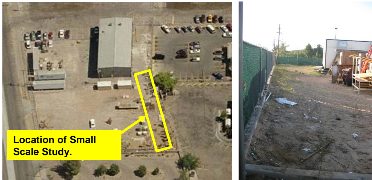
Figure 4.5 – Location of Asphalt Section at UTEP Facilities
