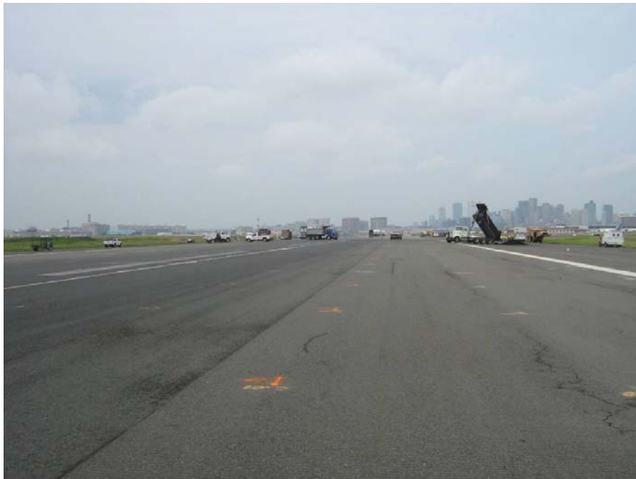
Figure 7.25 – Field Picture of Section 1
