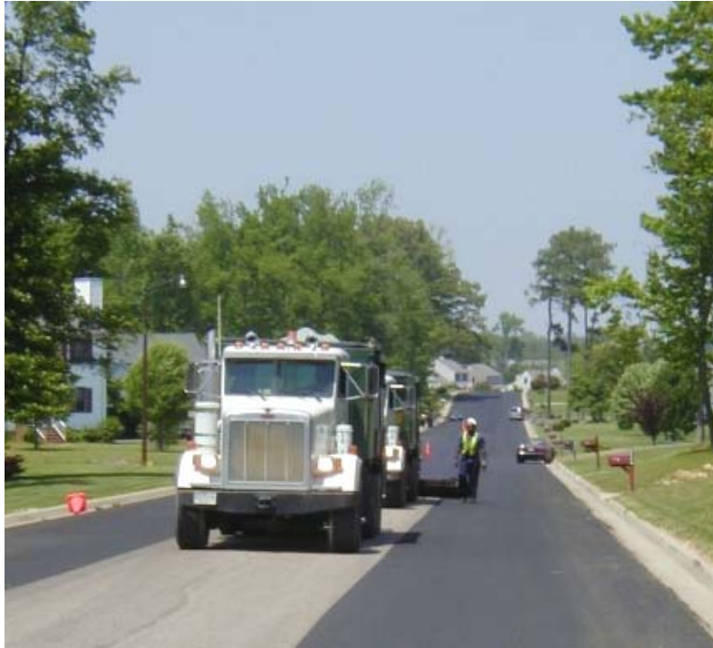
Figure 4.21 Slurry Seal Operation
