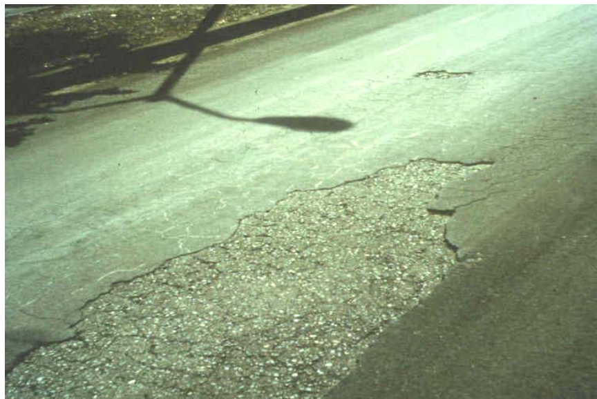
Figure 4.24 The Effect of Placing Slurry Seal on a Dirty Surface
