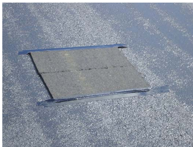
Figure 4.19 Felt Pad Used to Verify Application Rate
