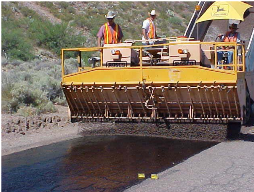
Figure 4.38 Self-Propelled Mechanical Distributor
