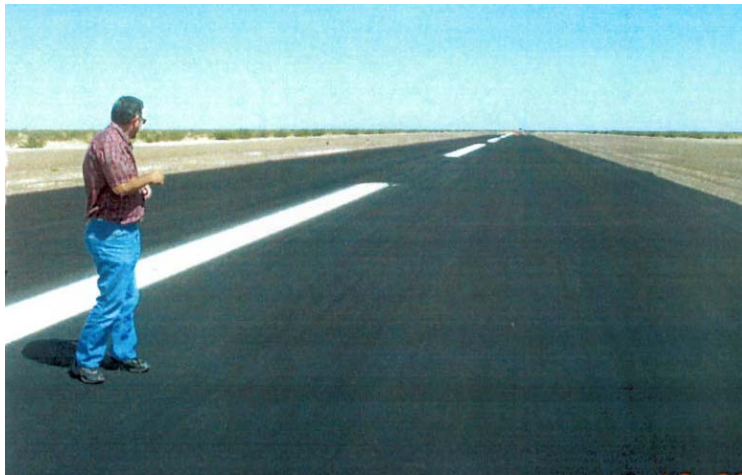
Figure 4.45 Completed Cape Seal at Yuma International Airport
