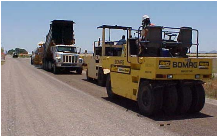
Figure 4.40 Pneumatic Roller Rolling a Chip Seal
