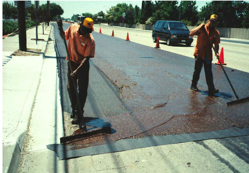
Figure 4.28 Starting from Roofing Felt
