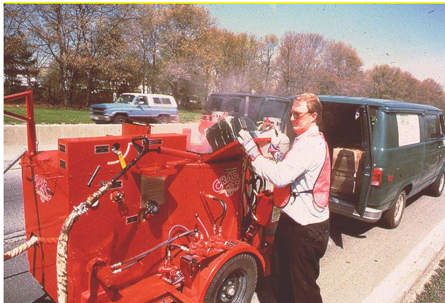
Figure 4.1 Hot-Sealant Machine
