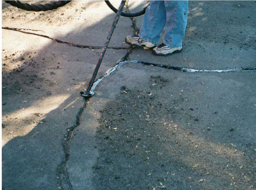
Figure 4.11 Placement of Sealant
