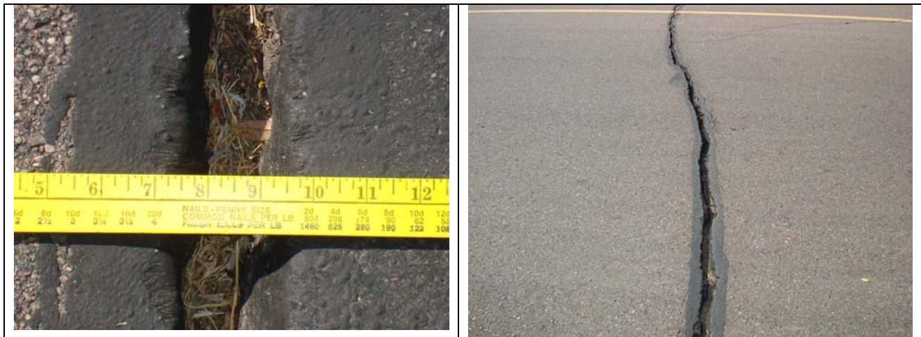
Figure 4.5 Medium Crack
