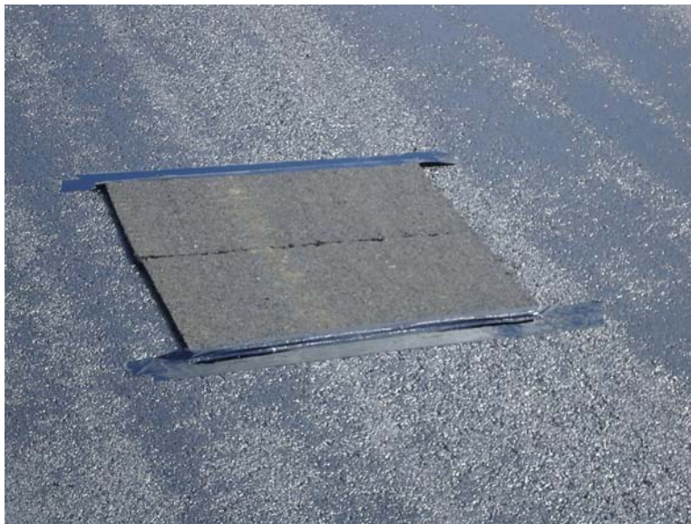
Figure 4.35 Fabric Being Used to Check Calibration of Distributor
