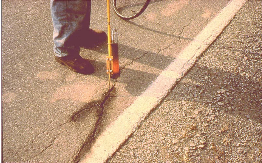
Figure 4.8 Using a Hot Air Lance to Dry a Crack
