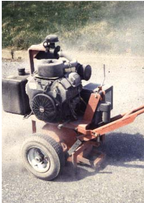
Figure 4.2 Router Being Used to Clean a Crack
