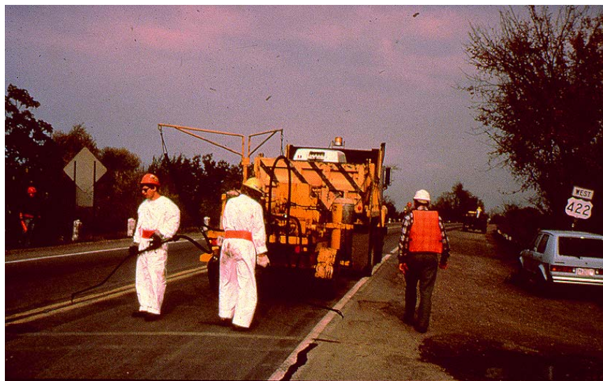
Figure 4.10 Sealing Cracks with Wand and Kettle
