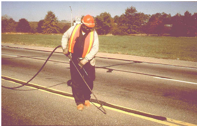
Figure 4.7 Using Air to Clean Out a Crack
