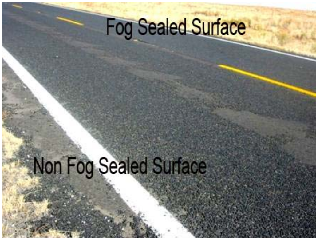
Figure 4.41 Effect of Fog Sealing on Performance of Chip Seal after Four Years
