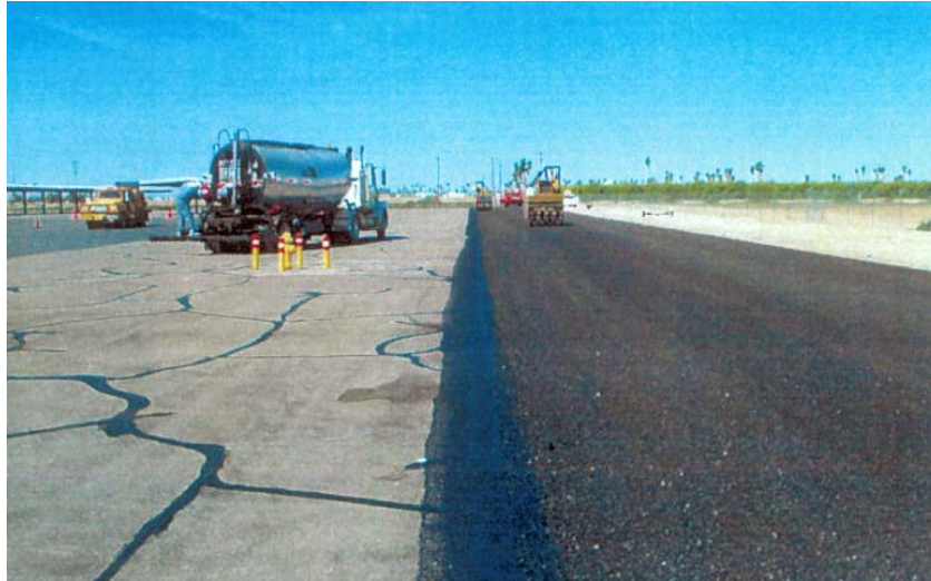
Figure 4.44 Cape Seal at Yuma International Airport
