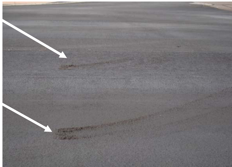
Figure 4.29 Initial Scuffing of Slurry Seal
