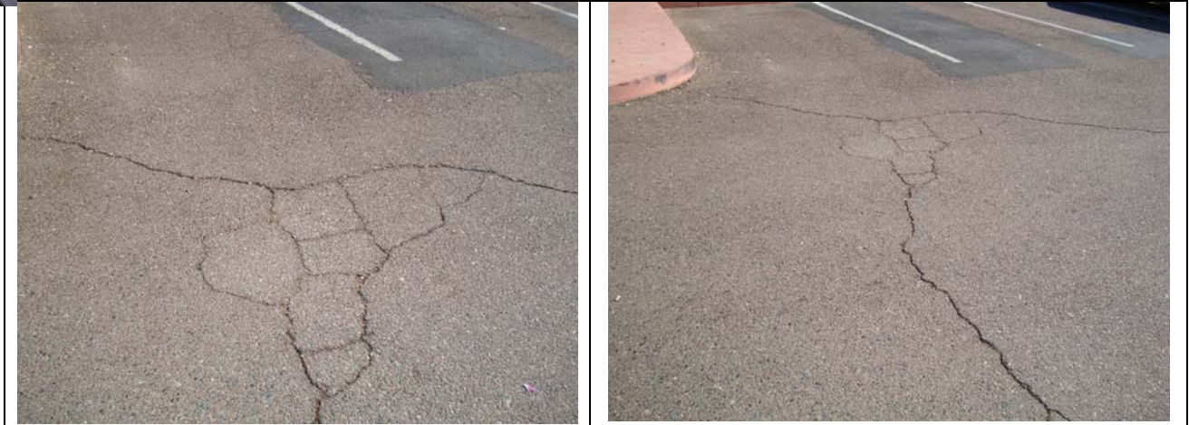
Figure 4.6 Multiple Cracks
