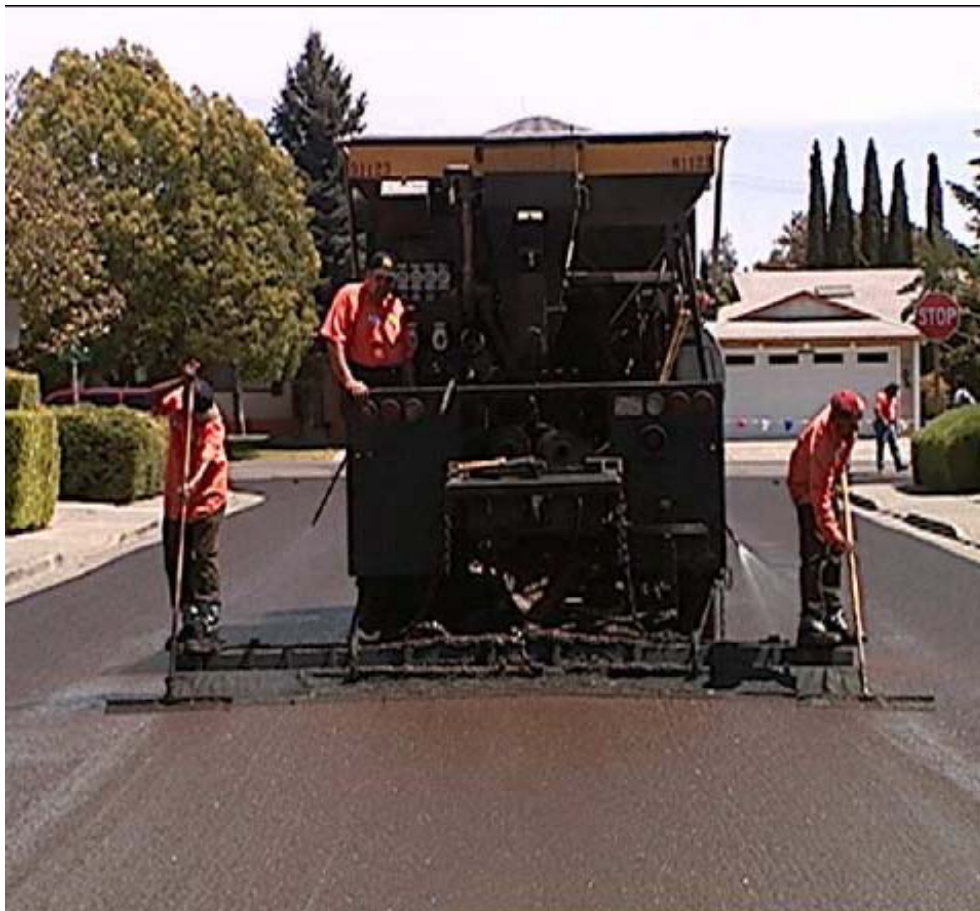
Figure 4.25 Slurry Seal Machine
