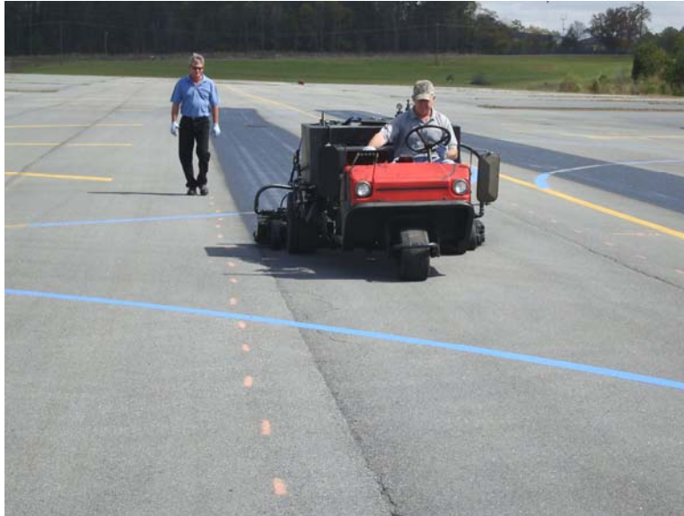
Figure 4.15 Spray-Applied Seal on an Army Airfield
