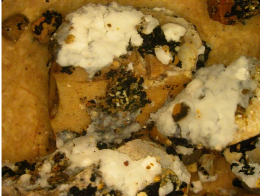
Figure 37. Severe Stripping of Uncompacted HMA at Conclusion of Dilatometer Test
