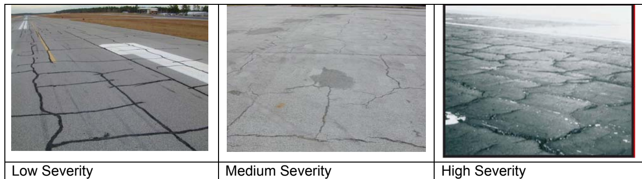
Figure 3-1 Block Cracking
