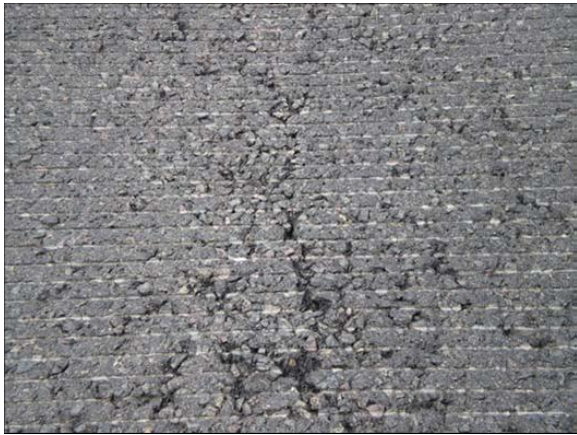
Figure B-20. Boston Logan Runway 06/27 near Taxiway C. Moderate severity raveling of the transverse grooved asphalt concrete surface.
