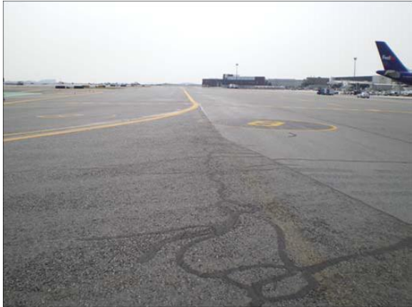
Figure B-11. US Airways Cargo area apron and south outer Taxiway K, Boston Logan Airport. Milled and overlaid with P-401 asphalt concrete in 2000. Note the cracked, segregated and raveled surface.
