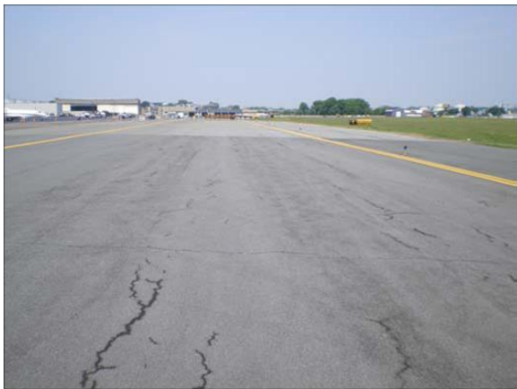
Figure B-24. Boston Logan Taxiway K between Taxiway N and Taxiway Z. Microsurfacing was placed over the raveled and stripped asphalt concrete.
