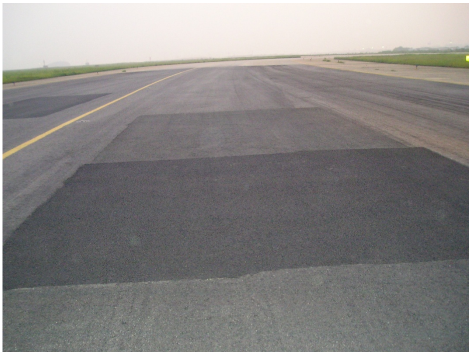
FIGURE 3.4 2005 Repair on Runway Extension.
