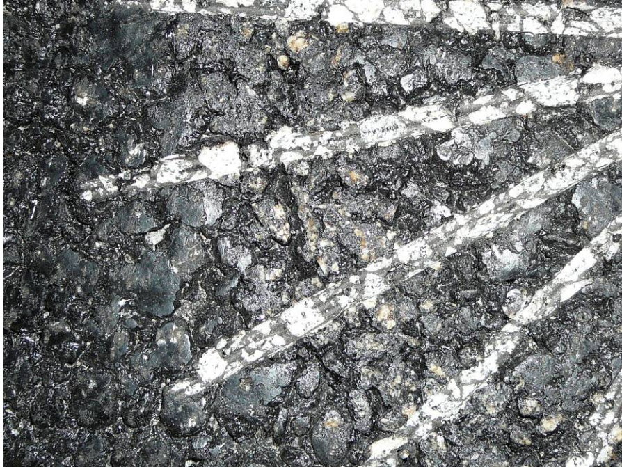
FIGURE 4.21 Close-up of Groove after 20,000 Revolutions.
