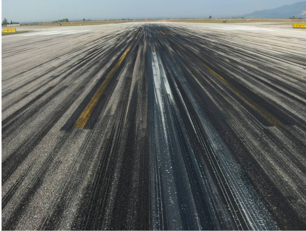
Figure 3.11 Rubber Build-Up at Aviano.
