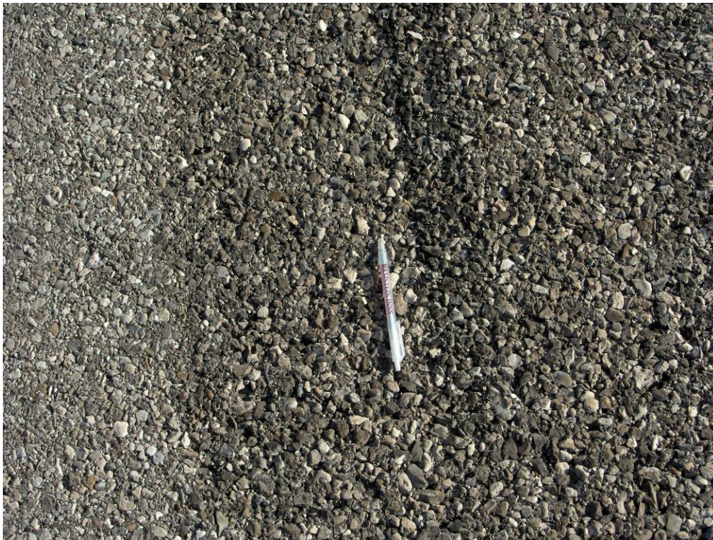
FIGURE 3.12 Differences in Surface Texture between Paving Lanes.
