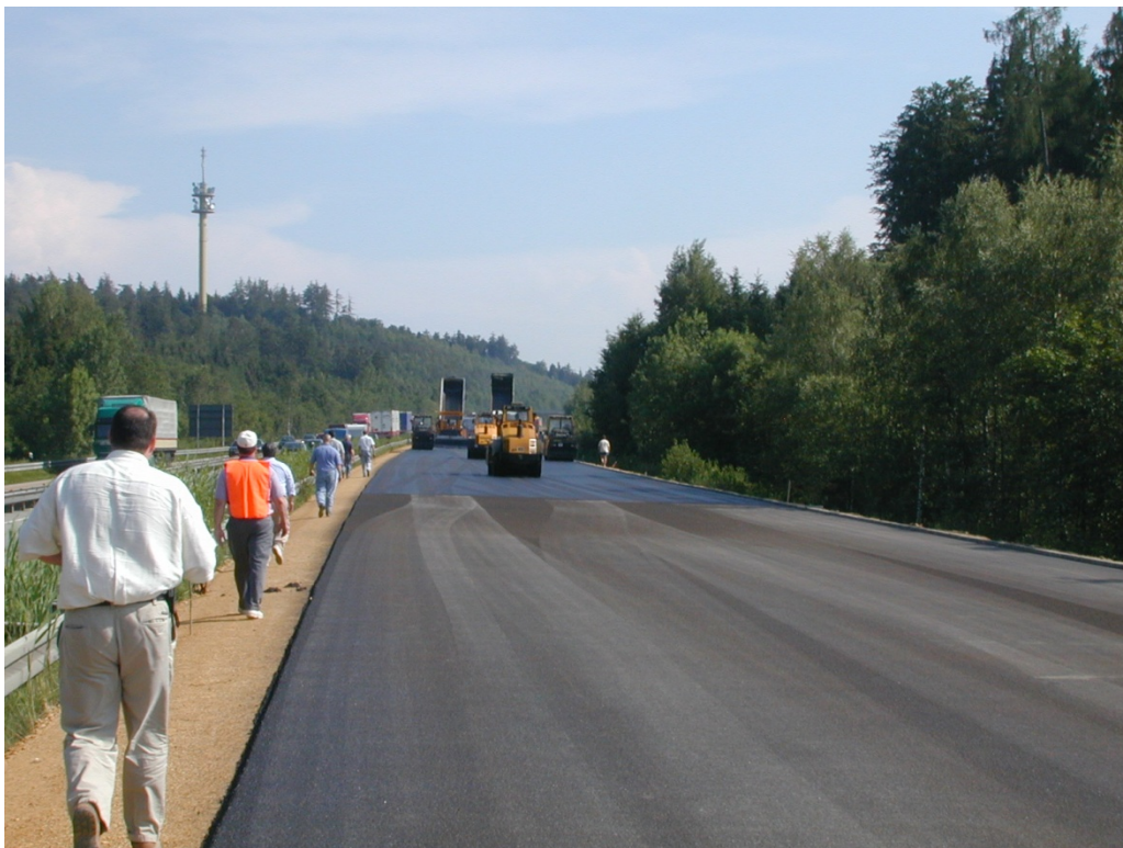
FIGURE 2.9 Grittied (Foreground) and Non-Grittied SMA Surface.
