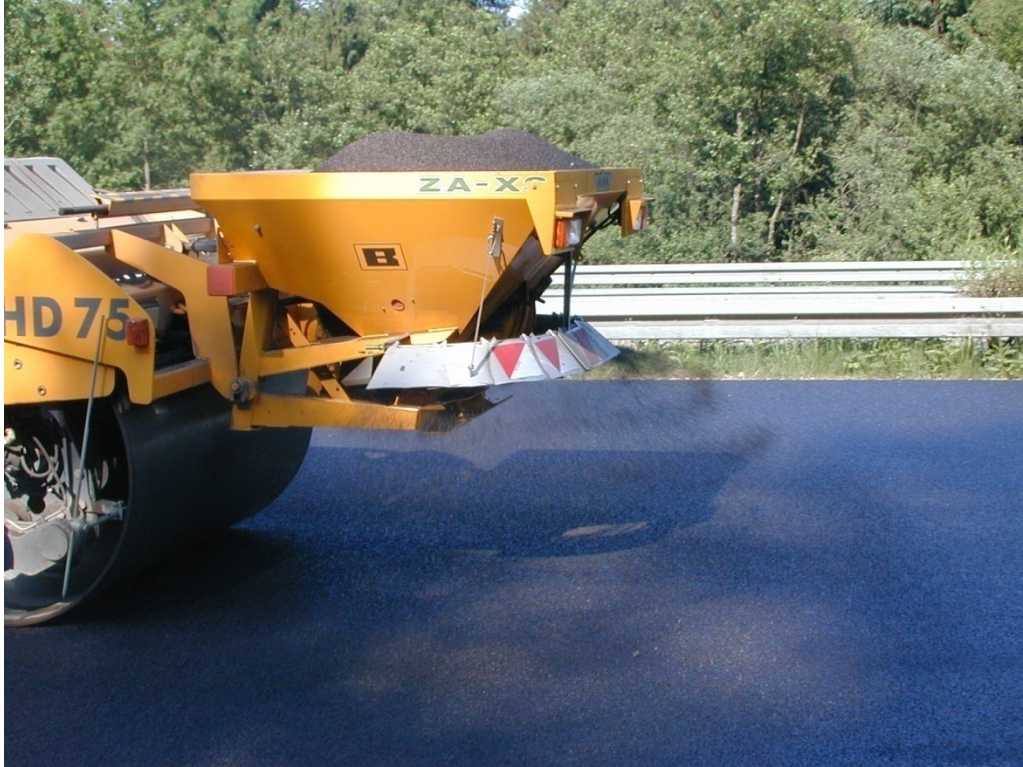
FIGURE 2.8 Application of Grit to SMA on Autobahn 3, near Passau, Germany.
