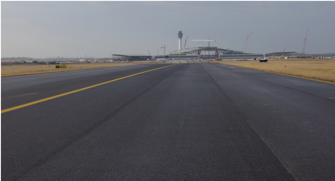
FIGURE 3.15 Overview of Taxiway “H,” Indianapolis International Airport.
