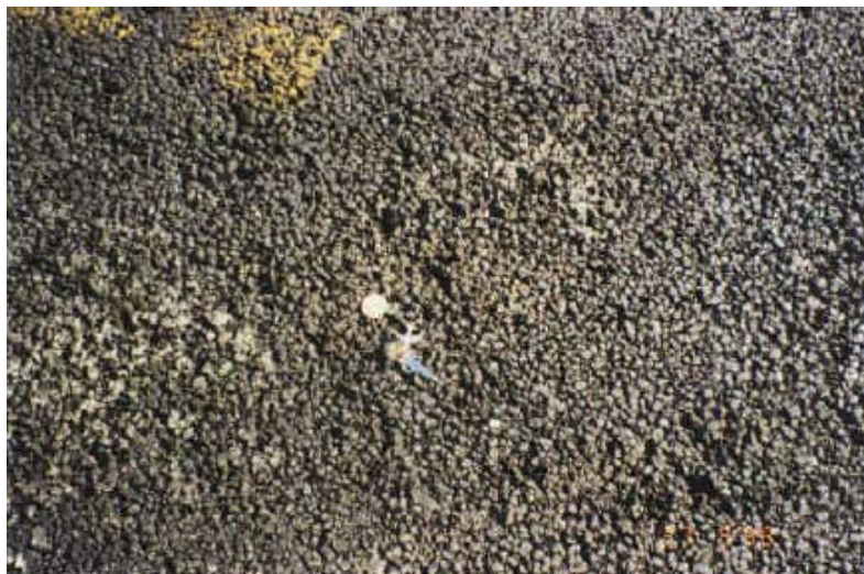
FIGURE 3.1 Typical Open Texture Area at Sydney International Airport.
