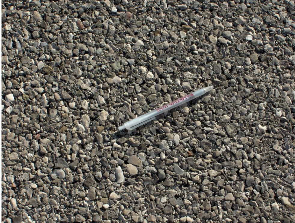
FIGURE 3.10 Typical SMA Surface Texture at Aviano.
