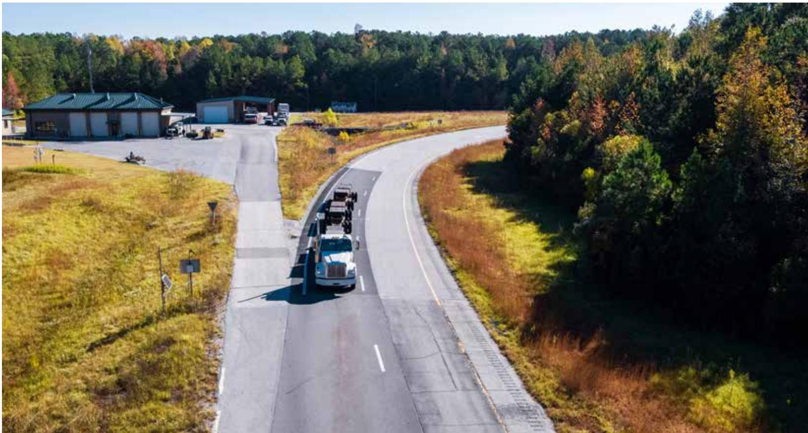
**NCAT's Test Track unites real-world pavement construction with live heavy trafficking, allowing researchers to quickly analyze and implement findings.**
